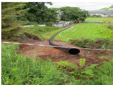
9 Culvert pipe within Kintyre Park
