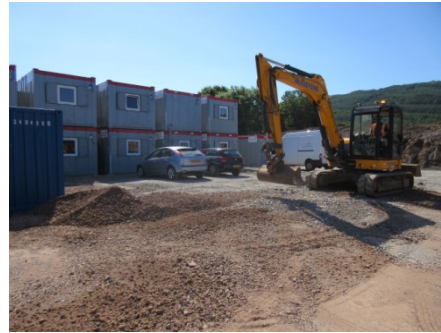
4 Site compound offices
