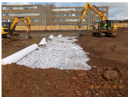
14 Preparatory ground works
