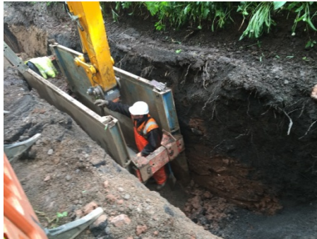
5 Culvert works taking place in the Cutting
