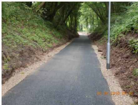
7 Completed works & new lighting in the Cutting
