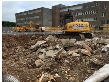
12b Music Block demolition
