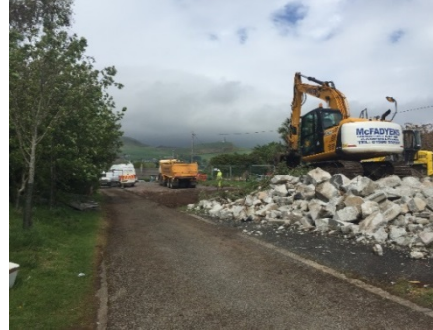
11b Demolition of the Boat Shed
