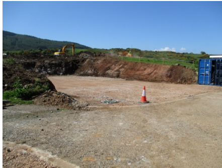
3 Site compound area
