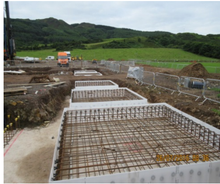
15b Installation of pad foundation reinforcement with Pecaform.
