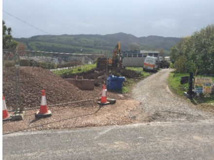
11a Site access showing Boat Shed in the background
