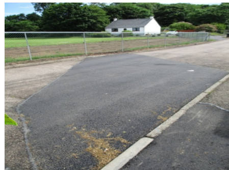
8 Re-instatement of Limecraigs Road
