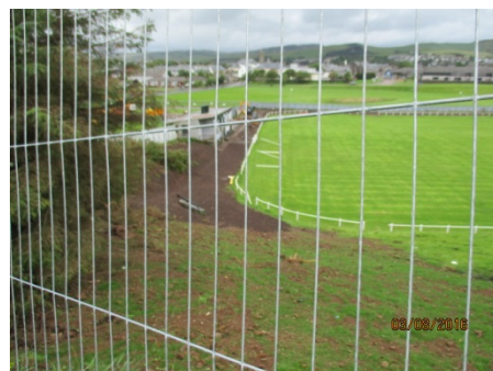
10 Kintyre Park re-instated following culvert works
