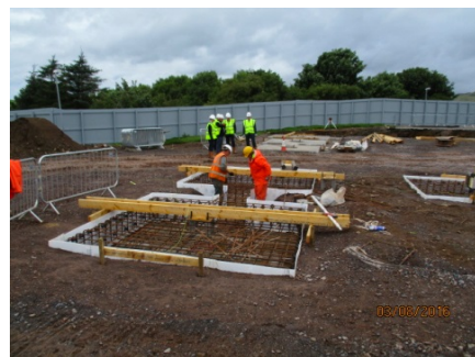
15a Preparing Concrete Foundations
