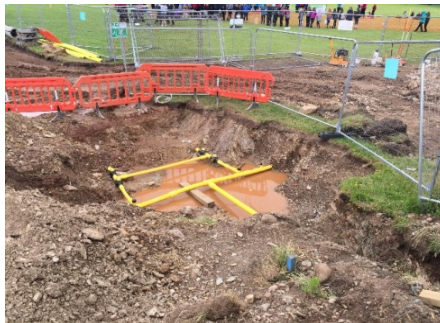
13a New Gas main installed
